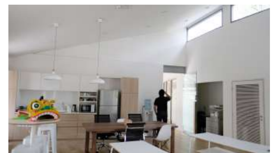
Daylit teacher lounge via clerestory opening
